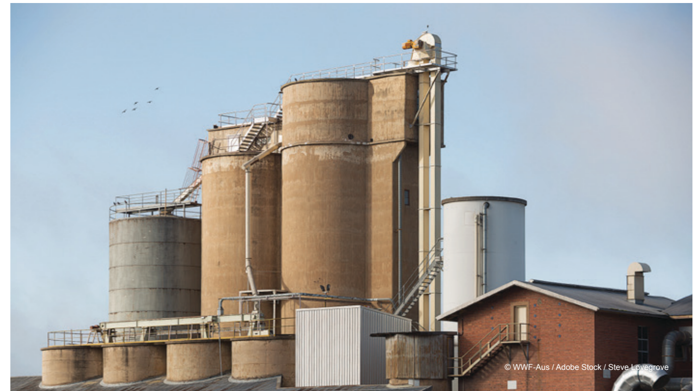
Through new investment, old fertiliser factories can be adapted to use renewable hydrogen.
